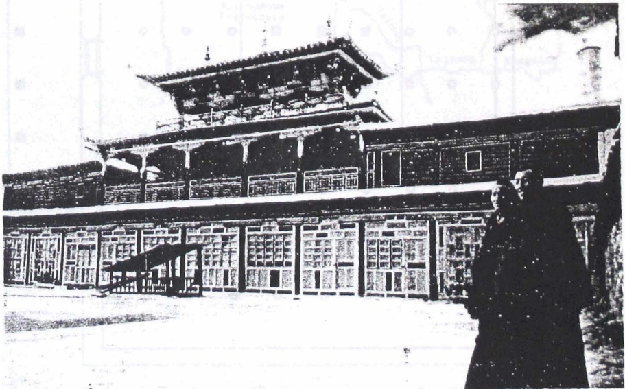
Structure above the main roof of the Assembly Hall
